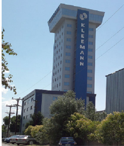
Fig. 8.75 Kleemann tower built in 2011
