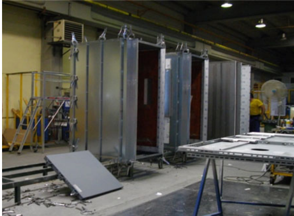
Fig. 8.102 Work site for cabin assembly (Danaktisi 2010)
