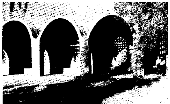
81. Vaults in the New Gourna Marketplace
