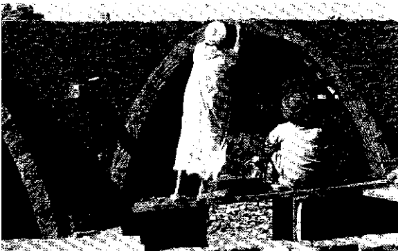
17. Masons insert dry packing in the interstices
