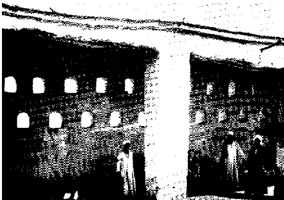
49. Loggia wall with openings to the windward side
