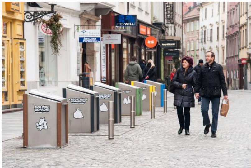
Figure 8: Underground collection points in central city and neighbouring areas, in Ljubljana (JP VOKA SNAGA)
