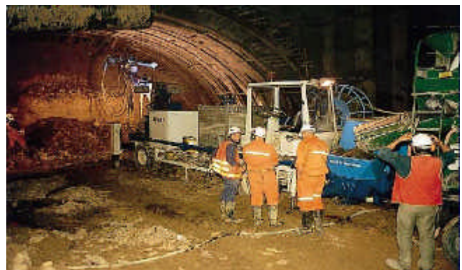
Figure 6: Use robotic spraying for higher quality sprayed concrete
