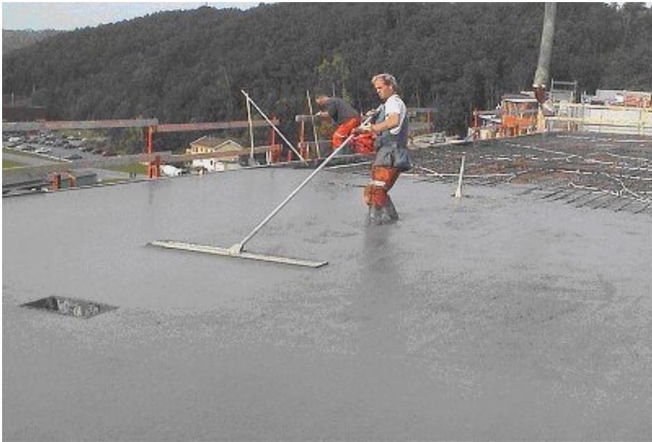
Figure 11.1 Levelling SCC with a skip float
