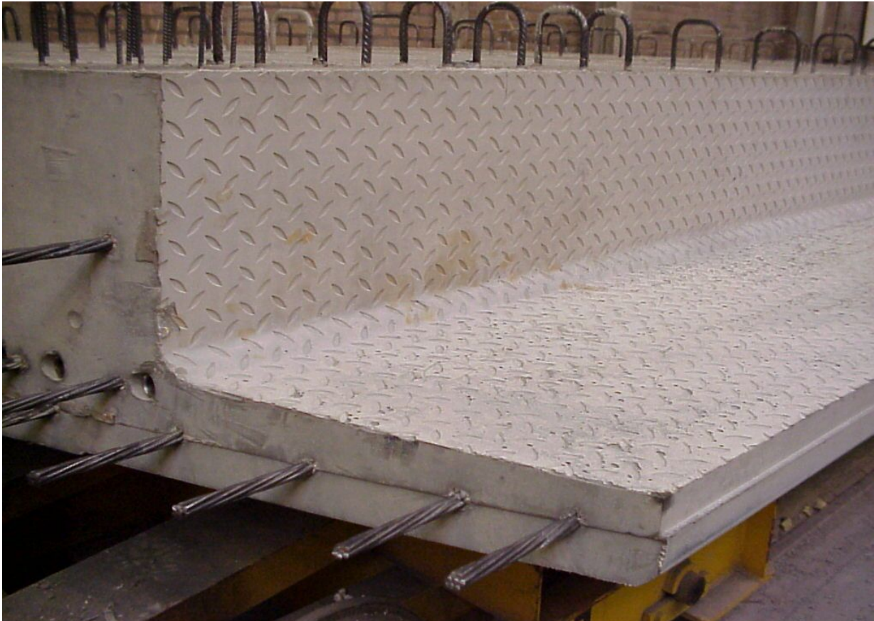
Figure 5.1: Surface detail on precast element with SCC filling under the formwork.
