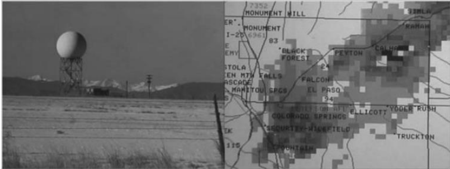
National Weather Service WSR-88D Doppler radar at Pueblo County, Colorado, USA and example of Storm Total Precipitation output ( http://www.crh.noaa.gov/pub/?n=/radar_about.php )
