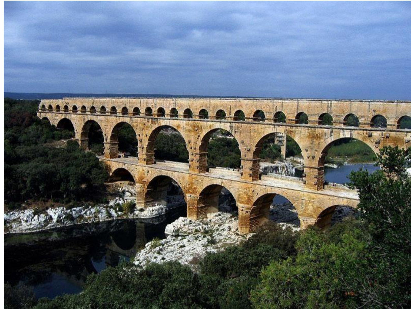
The Pont du Gard is an ancient Roman aqueduct bridge built in the first century AD to carry water over 50 km (31 mi) to the Roman colony of Nemausus (Nîmes)
