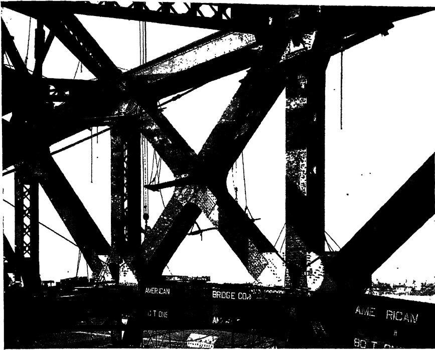
STEEL CONSTRUCTION. THE STEEL CORPORATION
