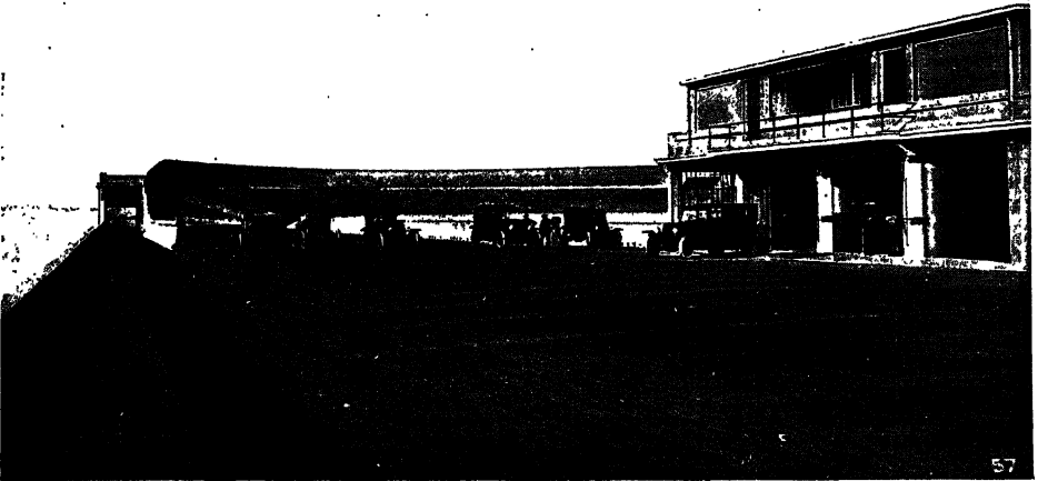
THE "FIAT" WORKSHOPS AT TURIN WITH THE TESTING TRACK ON THE ROOF 287
