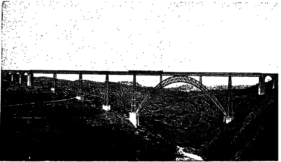
PONT DE GARABIT Designed by Eiffel the engineer.
