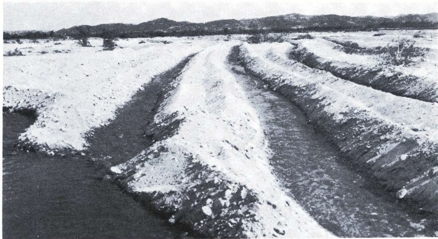
Fig. 13.4 Spreading ditches in Tujunga Wash, Los Angeles, California (courtesy City of Los Angeles Department of Water and Power).
