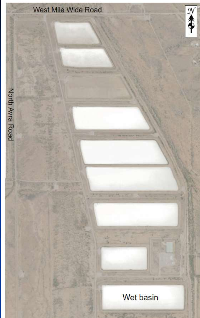
Fig. 15.12 Aerial photographs of the Central Avra Storage and Recovery Project located near Tucson, Arizona (May 2015; Source U.S. Geological Survey)
