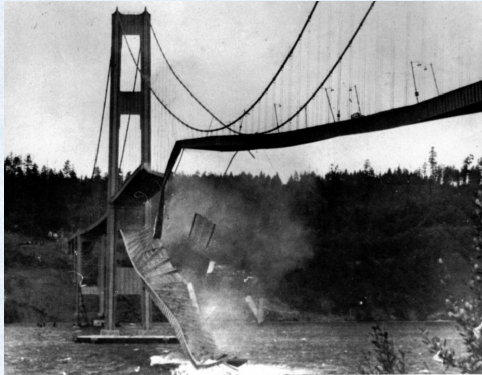
Collapse of the Tacoma Narrows bridge in 1940.
