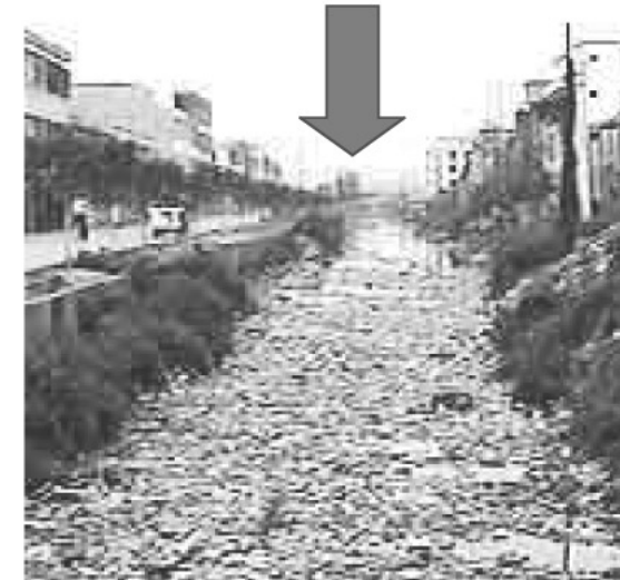
Guiya, China, irrigation canal – town stream nearly choked with e-waste.
