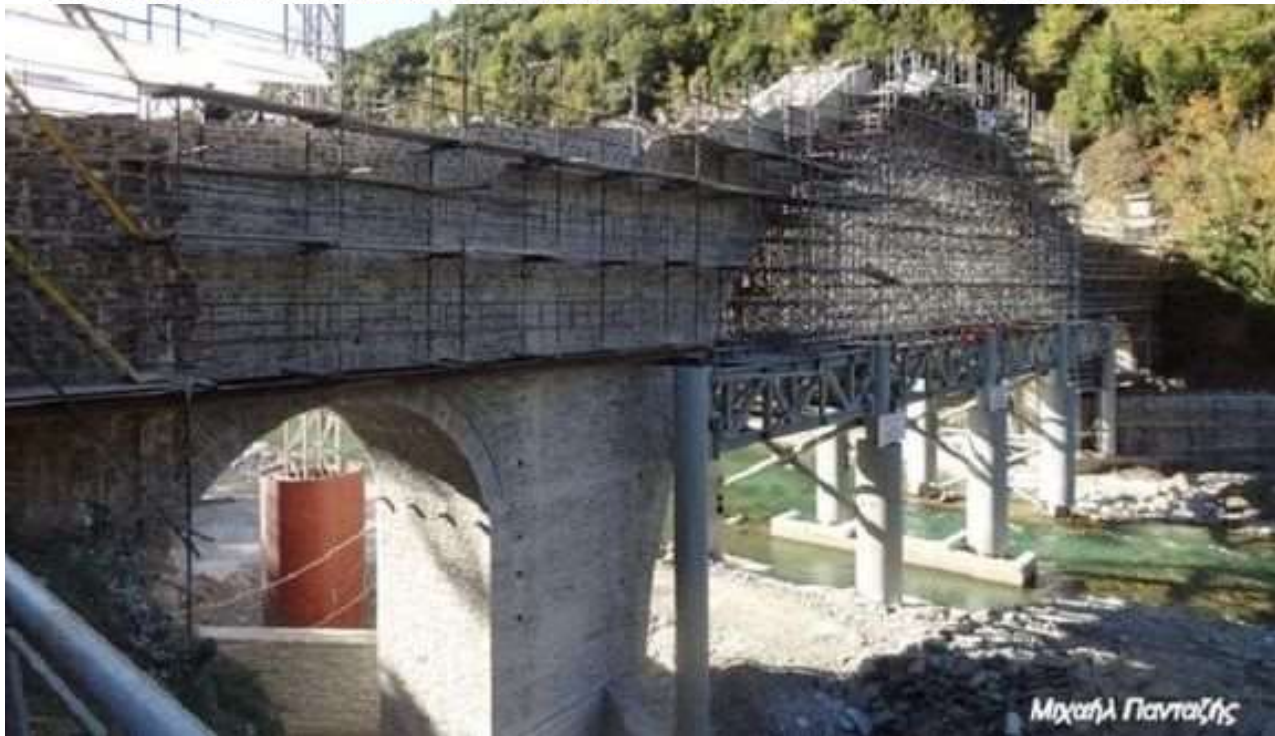
Fig 8: Basic elements of arch bridge construction. The arch is constructed symmetrically over a temporary formwork. Note that the arrangement of the stones differs entirely between the arch and the abutment. Stones of
