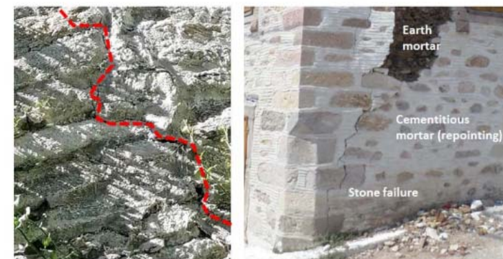
Figure 12: A zig-zag crack through the joint mortar in the bridge (left). An example of implications of incompatible repointing mortar in a historic stone masonry building (right).
