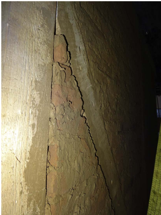
Fig. 42. Out of plane of the infill.
