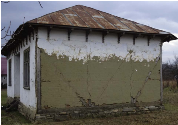
Fig. 12. Upper structure of the house (Fig. 9 was made after this house).
