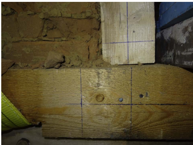
Fig. 38. Bottom marginal connection with small uplift.
