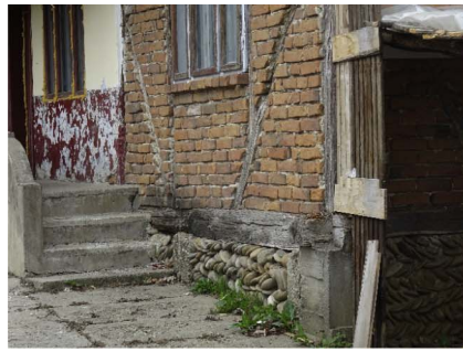
a. The foundations are made only from stone (river rocks)
