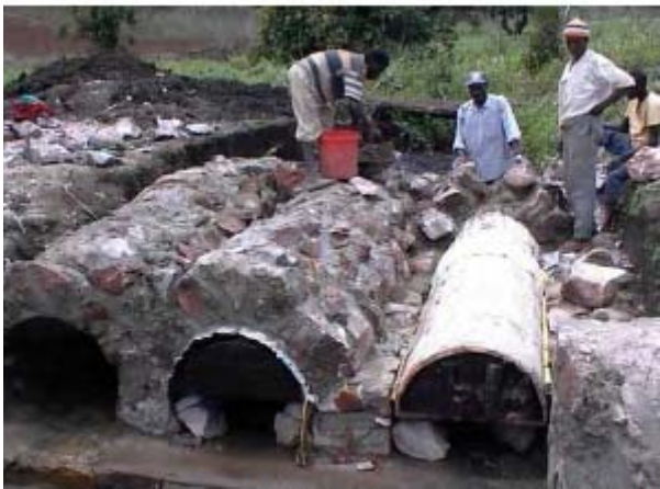
Fig 9: Construction of a multiple-arch culverts with stones found in the vicinity
