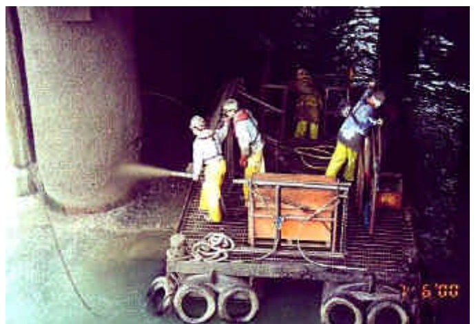
Figure 30 (Courtesy: Spraycon Ltd)
