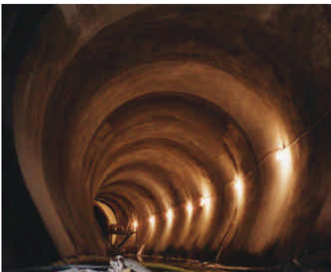
Figure 24: Screed and float finish permanent sprayed concrete tunnel
