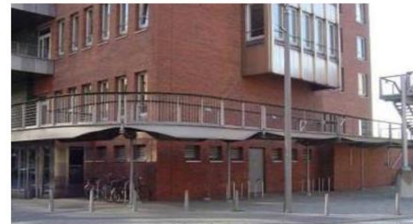
Figure 5.12 Example of dry proofing Hamburg, Germany
