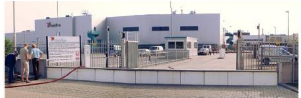
Figure 5.18 Permanent flood gate Meppel, The Netherlands Source: Floodbarrier.nl, 2011
