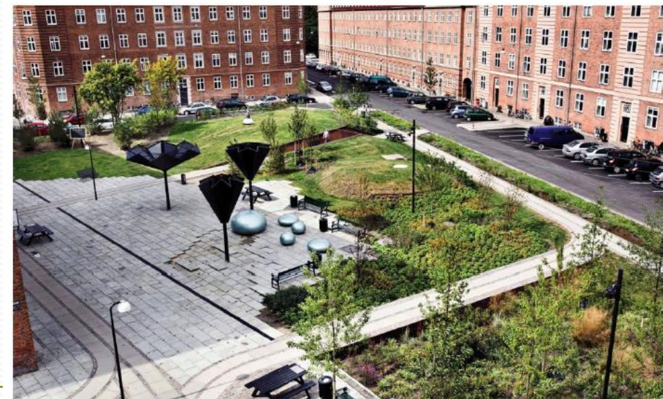
Figure 28. Tansinge Plads - square and a water retention basin, designed to hold back
