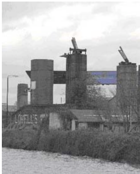
Fig. 3. Lovell's wharf – crane base in 2007 (now destroyed and replaced by apartments)
