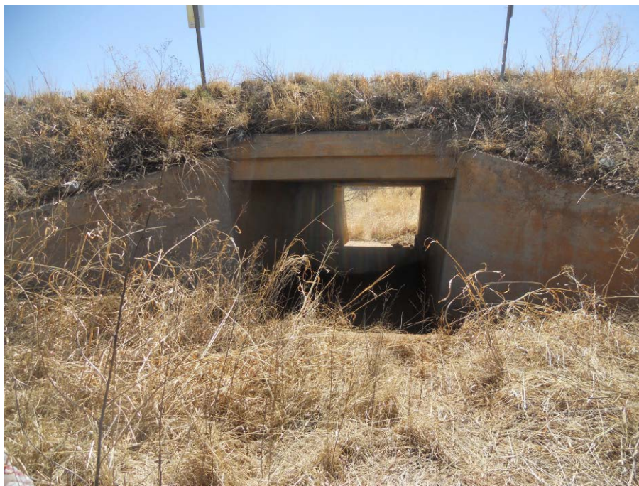
FIGURE 3. The box culvert at Site 1 (photograph by author).
