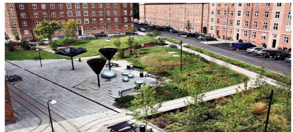
Figure 28. Tansinge Plads - square and a water retention basin, designed to hold back
