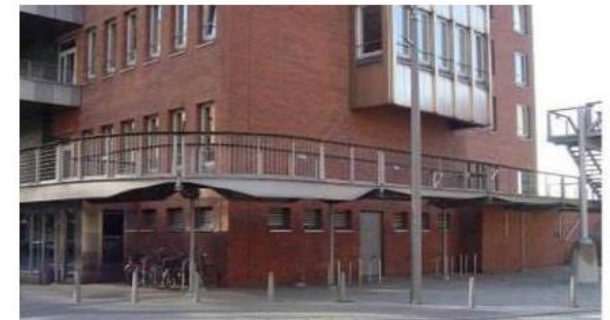
Figure 5.12 Example of dry proofing Hamburg, Germany
