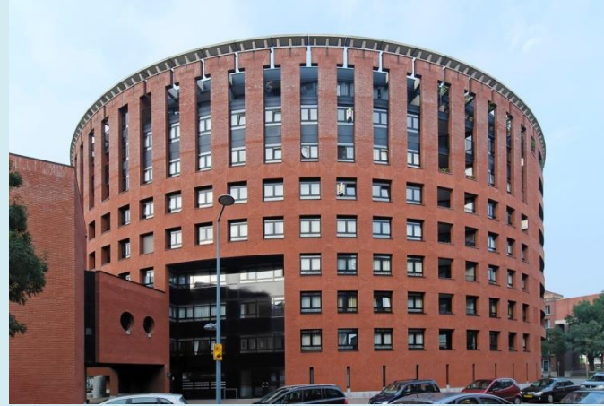
Mario Botta 2001-2008 Residential Building 'la vista' Belgium
