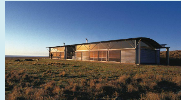
Glenn Murcutt 1984 Magney House
