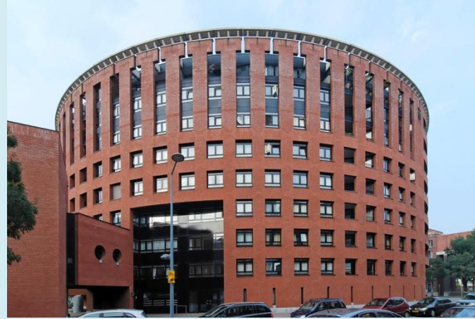
Mario Botta 2001-2008 Residential Building 'la vista' Belgium
