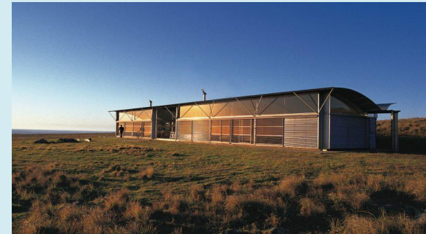
Glenn Murcutt 1984 Magney House
